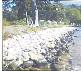
Rock Riprap – A very common hard-armor technique which consists of large rocks placed in the water and up the slope along the shoreline. Riprap should be lined with geotextile fabric to prevent wave action from sucking soils from behind rocks, causing slumpage. Glacial stone seawalls provide shoreline armoring while causing less damage to habitat and natural aesthetics.
